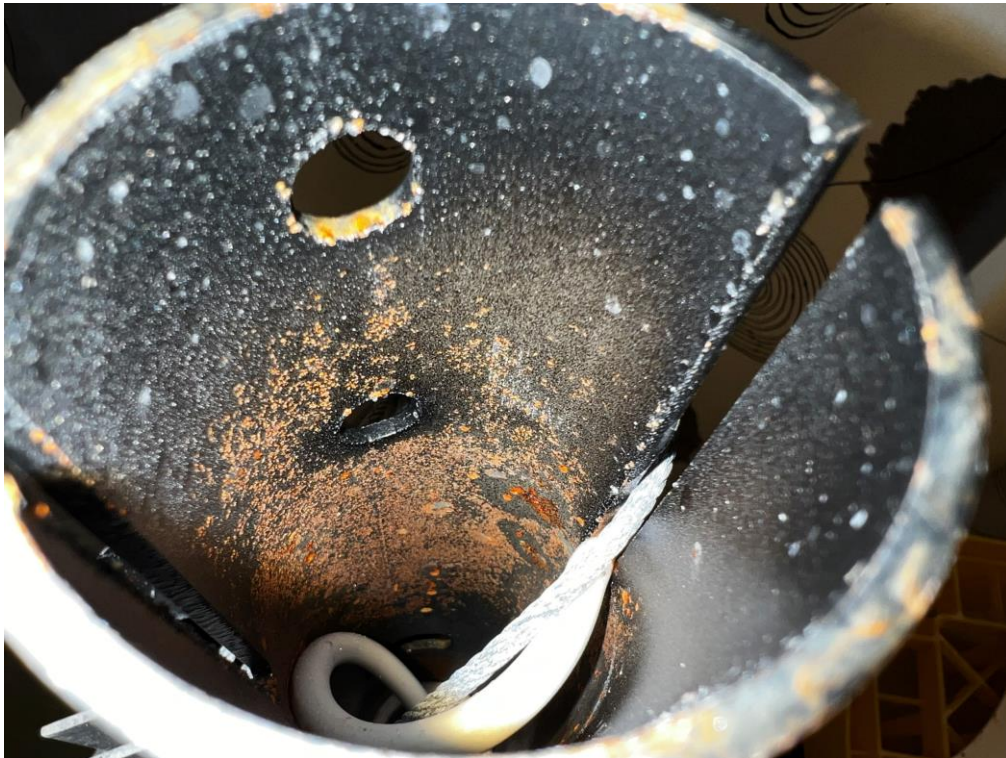
Photo 7 Visual inspection (fan). Corrosion on/inside fan extension tube.
